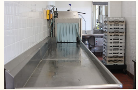
Clean, sanitized dishes leave this dishwasher at a piping 180 degrees and must cool before touching.
